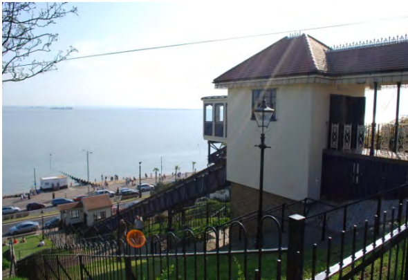
Cliff Lift, Western Esplanade (Central Seafront Policy Area)
